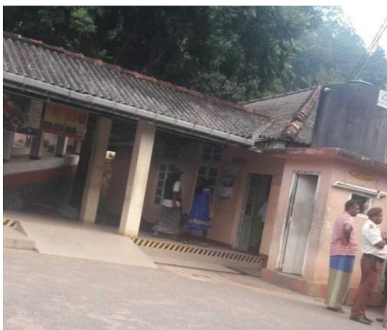
Asbestos roofing sheets & ceiling sheets to be removed during demolition at Kahawatta BH
