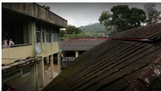
Asbestos roofing sheets & ceiling sheets to be removed during demolition at Kahawatta BH
