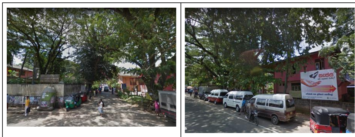
Figure 2. Photographs of Kahawatta BH
