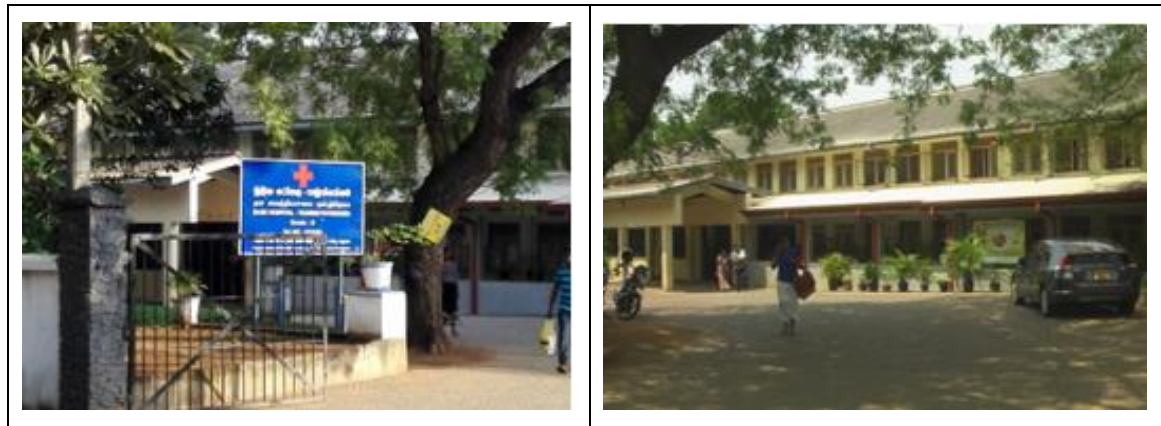
Figure 6. Photographs of Thambuththegama BH
