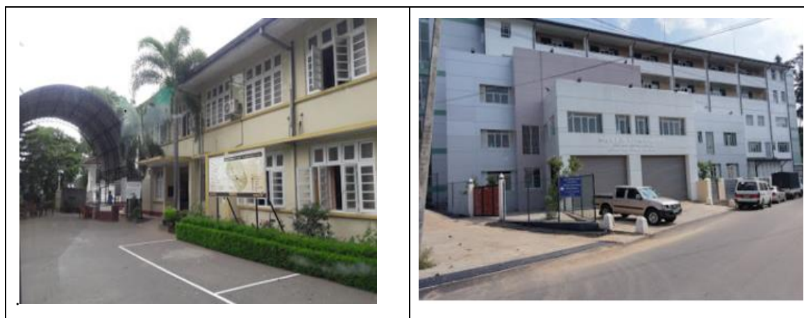
Figure 10. Photographs of Teldeniya BH
