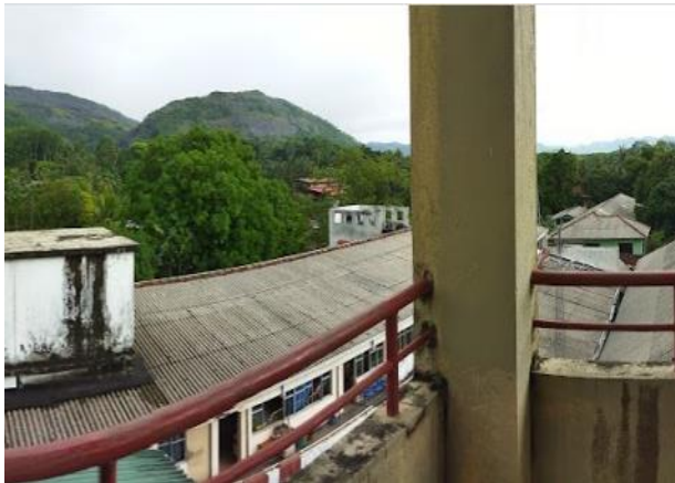
Asbestos roofing sheets & ceiling sheets at Medirigiriya BH
